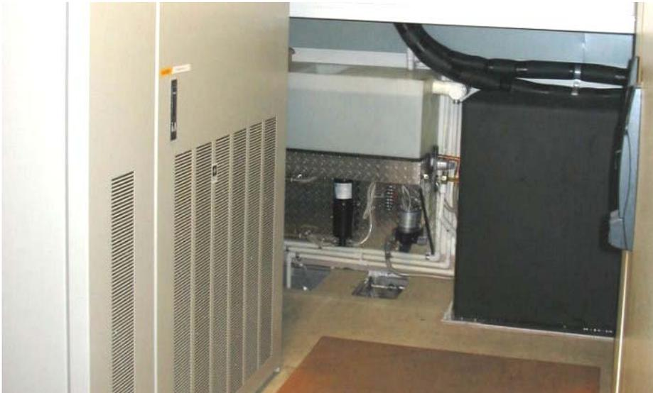
**Figure 42: Humidifier Tank**
