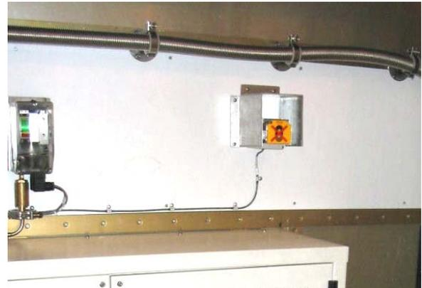
**Figure 17: Magnet Room E-Stop & Quench Buttons**
