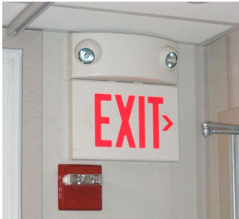
[Figure 51: Emergency Dual Beam Lighting](#)
