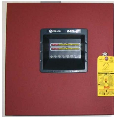
**Figure 26: Fire Alarm Control Panel**
