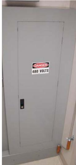
**Figure 34: 480V AC Electrical Panel**
