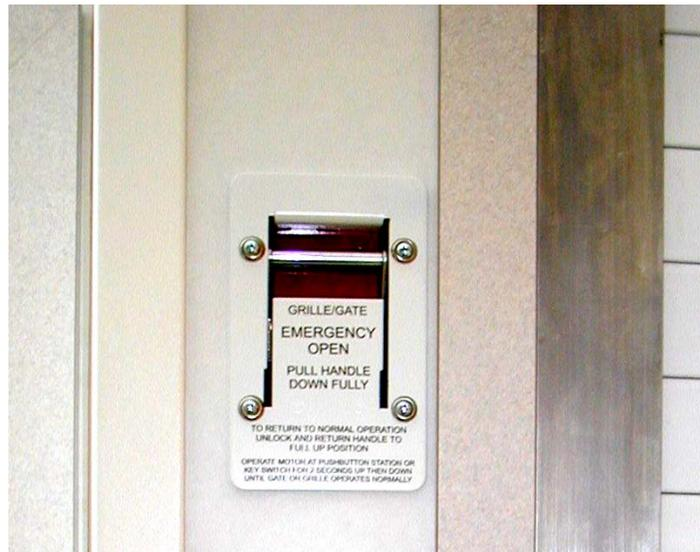
**Figure 31: Roll Door Emergency Release**
