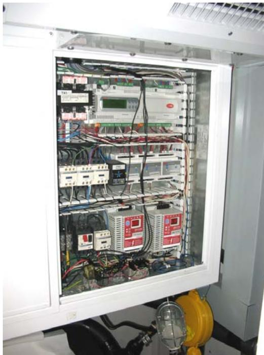
**Figure 40: A/C / Chiller Control Panel**
