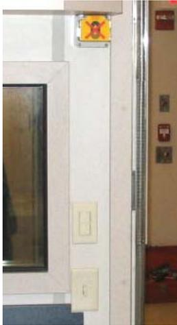
Scan Room Lighting and Magnet Quench Controls
