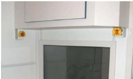
Scan Room E-Stop and Magnet Quench Controls
