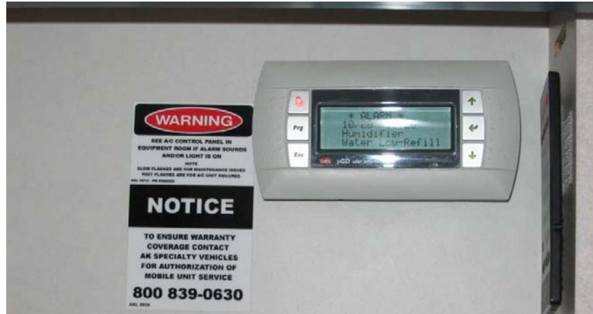
**Figure 41: A/C / Chiller Alarm Panel**
