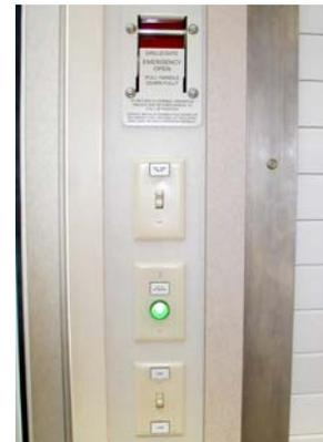
Roll Door Controls and Platform Lift "UP" light
