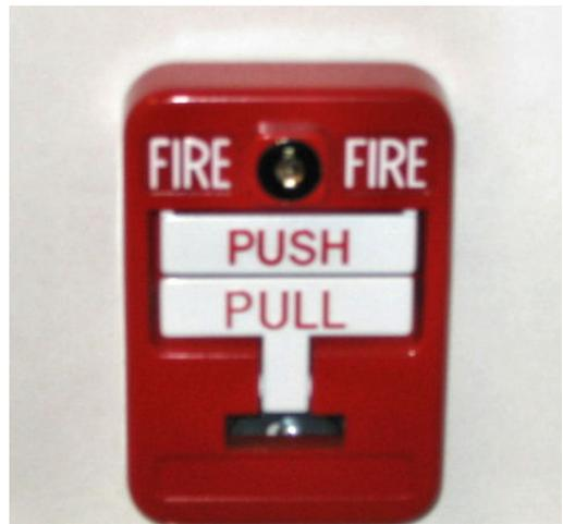
**Figure 27: Fire Alarm Pull Station**
